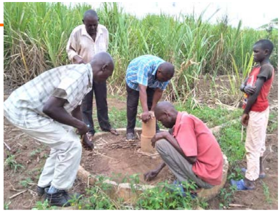
(An example of one of the many non-functional boreholes in Uganda. This perfectly drilled borehole in Kamuli was down for 13 years before being rehab'd by B.T.. Photo submitted by Harriet Naigaga )
